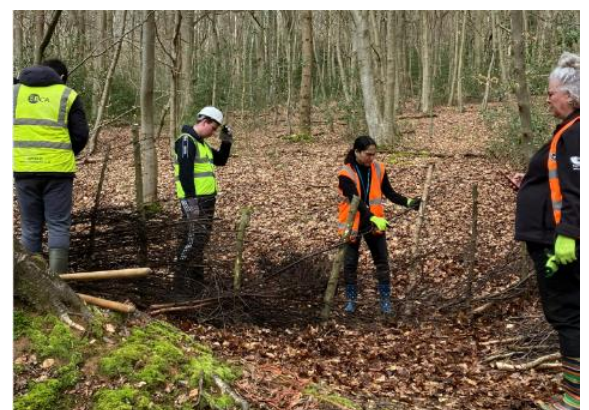
Image 8: Blocking a desire line, helped by staff and students from Berkshire College of Agriculture.
